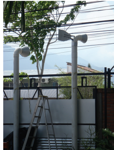
Figure 18 Set-up windward facing pipes.
